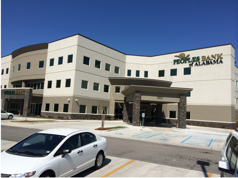
Photo 1 People's Bank of Alabama, home office, Cullman, Alabama, is located in a refurbished former medical arts building.
