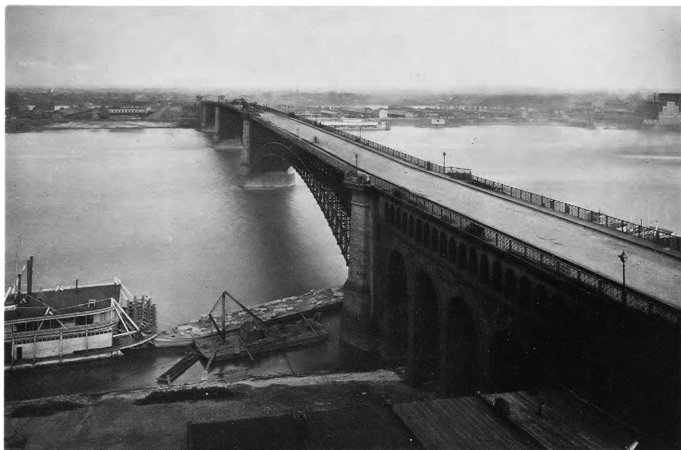
Eads Bridge at St. Louis (1880)
